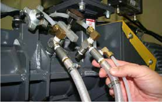
Air assisted jet assembly removed from the mixing chamber for physical calibration.
