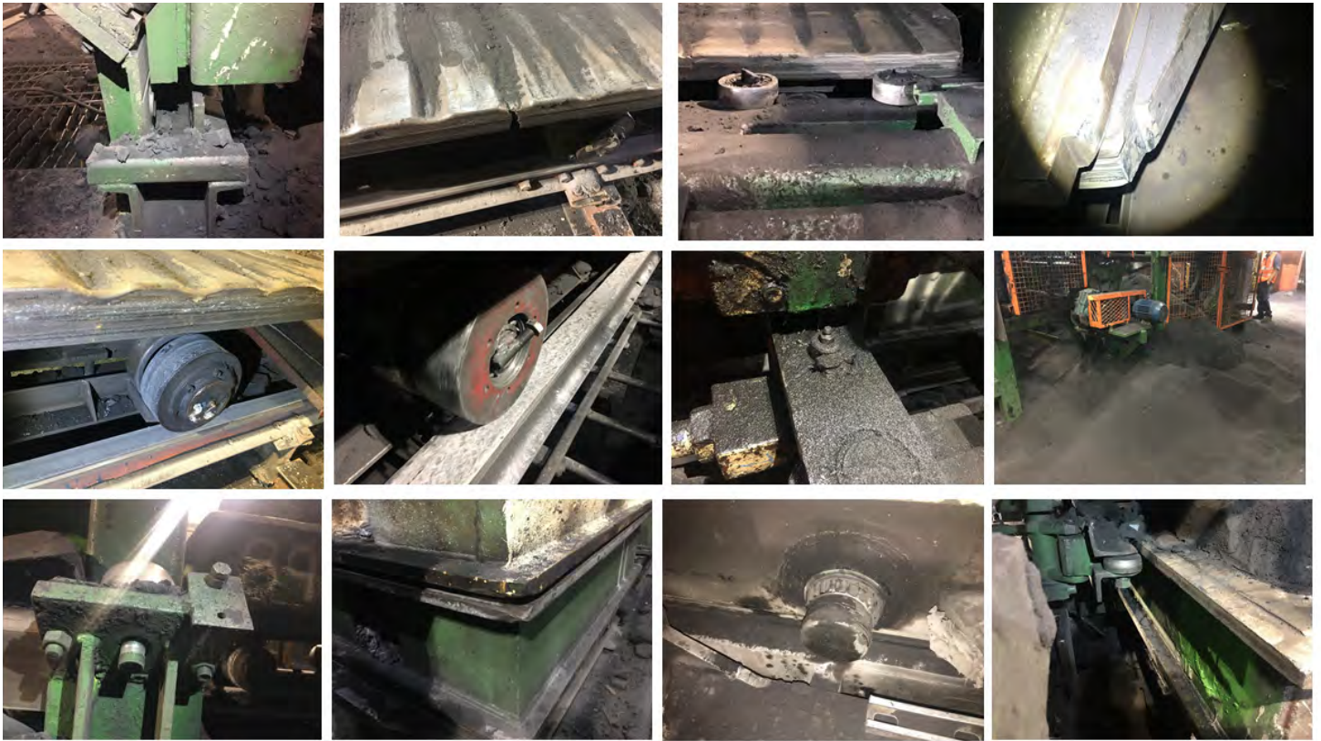
Above is an example photo gallery of damaged or nearing damaged devices that a professional service technician can identify along with corrective actions.
